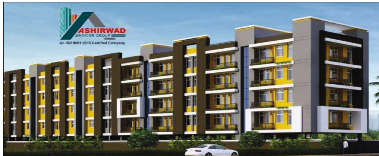
ASHIRWAD SIDDHI VINAYAK, BHOGIPUR, PATNA ON COMPLETION
